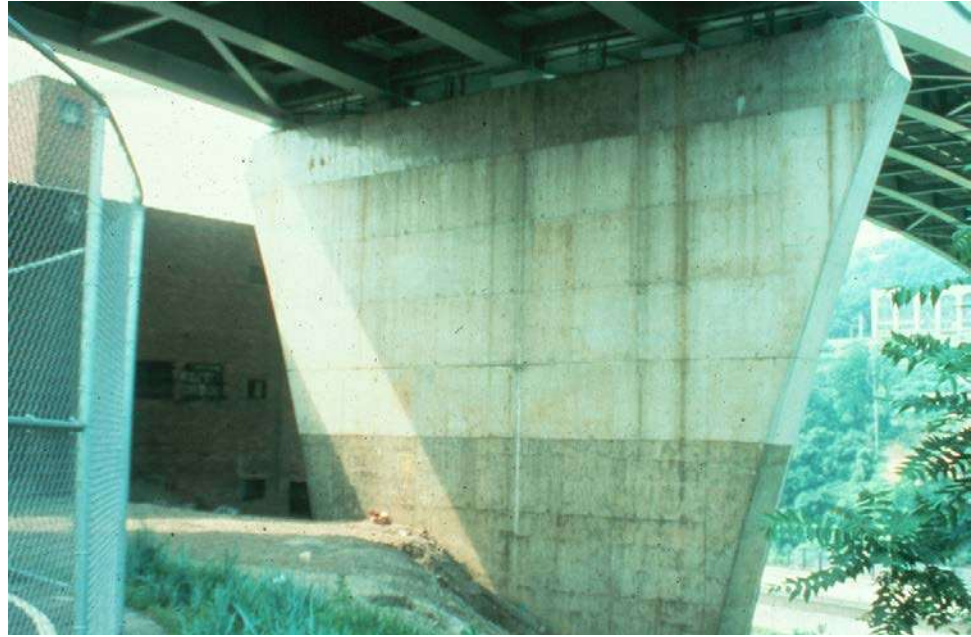
Figure 6.2.32 Anti-Graffiti Coating on Lower Area of Bridge Piers
