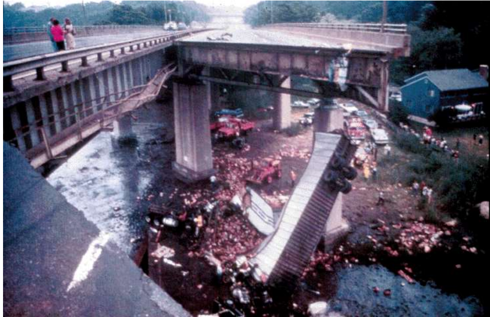
Figure 6.4.2 Mianus River Bridge Collapse
