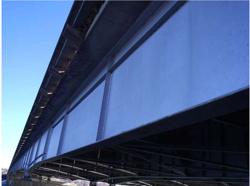
Figure 6.3.4 Welded I-Girder
