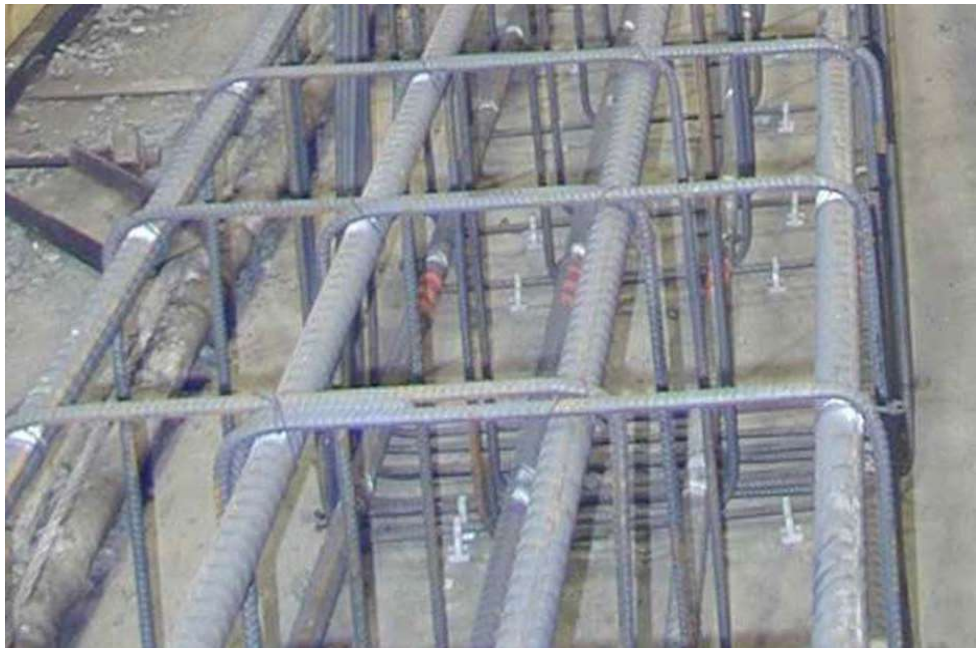
Figure 6.3.5 Steel Reinforcement Bars
