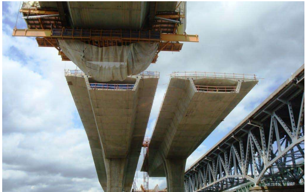
Figure 6.2.10 Post-tensioned Concrete Box Girders
