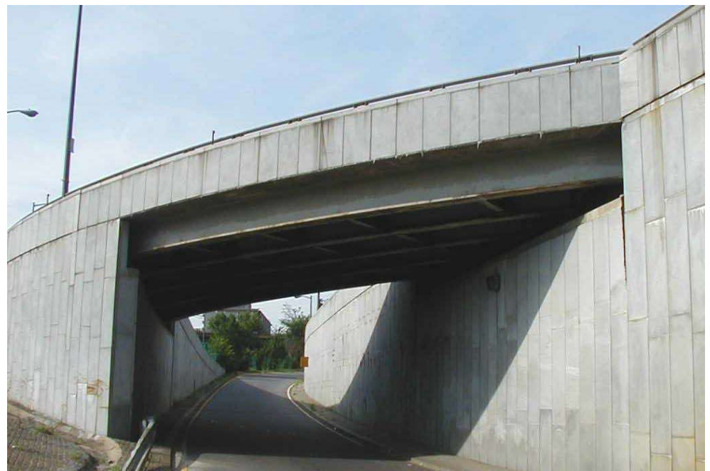
Figure 6.3.7 Rolled Beams
