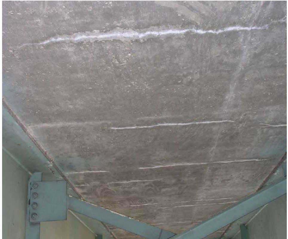
Figure 6.2.17 Transverse Cracks
