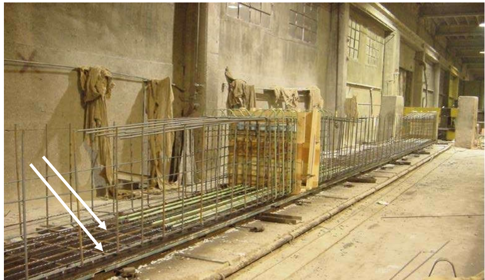
Figure 6.3.1 Prestressing Strands for a Box Beam
