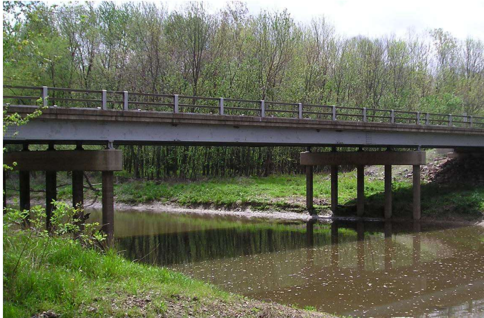
Figure 6.4.5 Structurally Redundant Continuous Span Bridge
