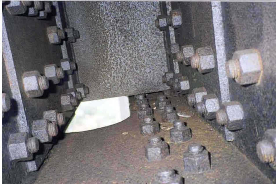
Figure 6.3.30 Black – Non-protective Oxide
