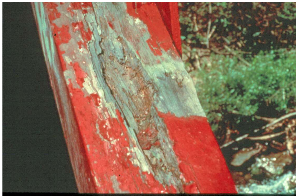
Figure 6.1.8 Decay of Wood by Fungi
