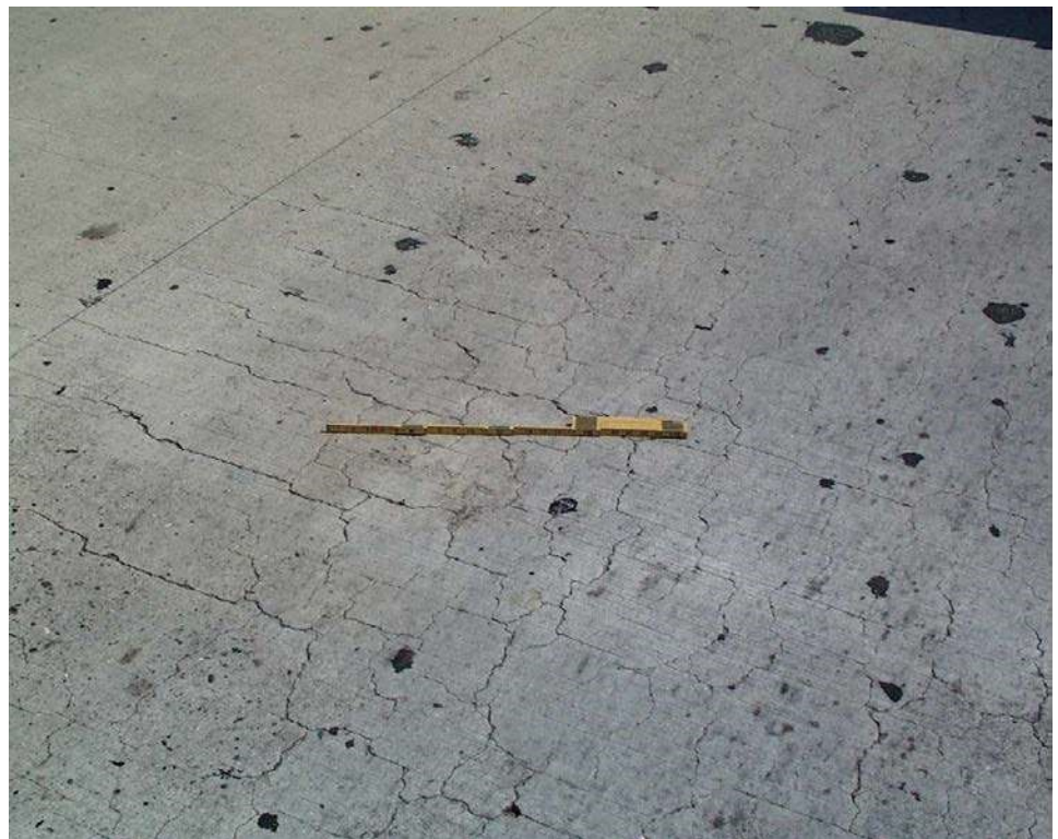
Figure 6.2.16 Shrinkage Cracks
