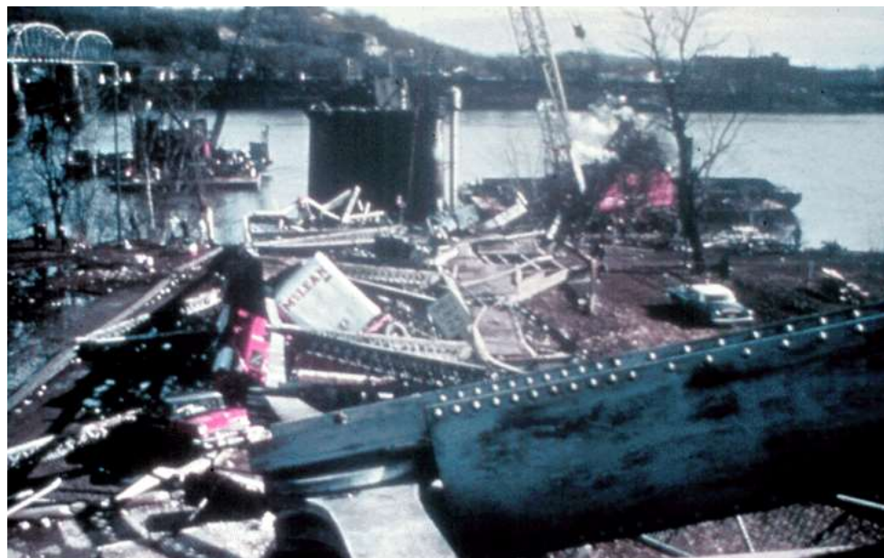
Figure 6.4.1 Silver Bridge Collapse
