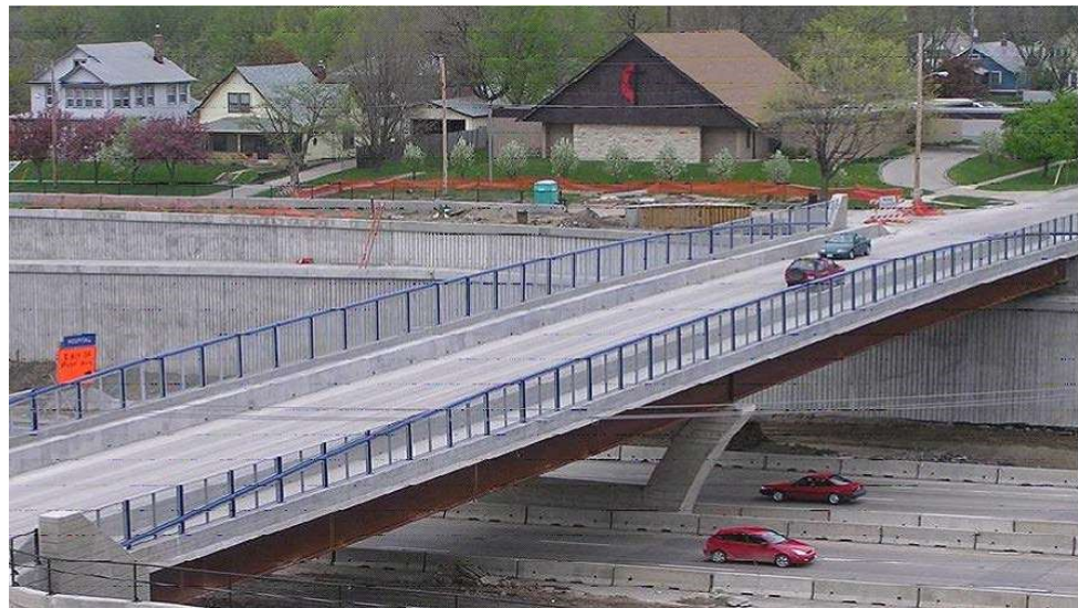
Figure 6.3.9 High Performance Steel Bridge
