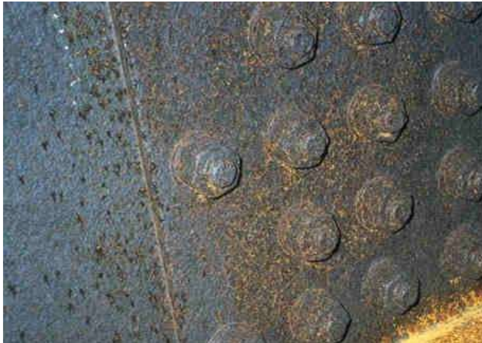
Figure 6.3.29 Chocolate Brown to Purple Brown - Fully Developed Oxide Film
