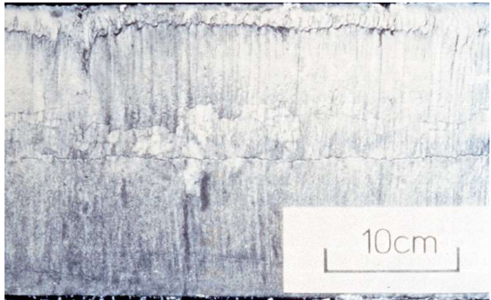
Figure 6.4.18 Exposed Lamination in Steel Slab
