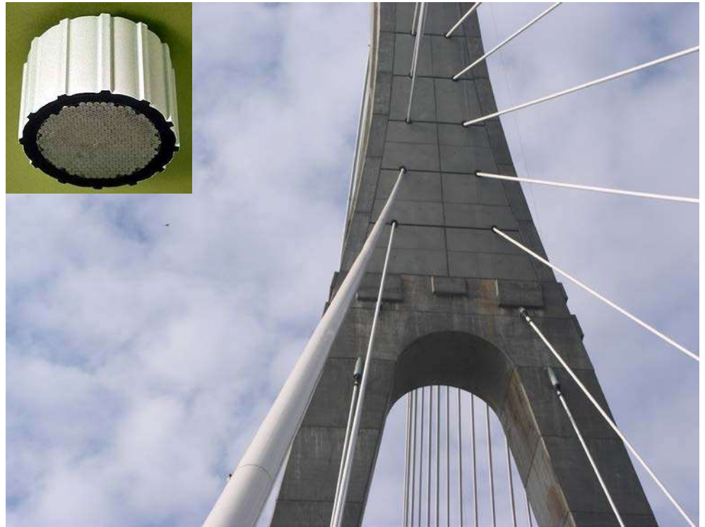
Figure 6.3.2 Steel Cables with Close-up of Cable Cross-Section
