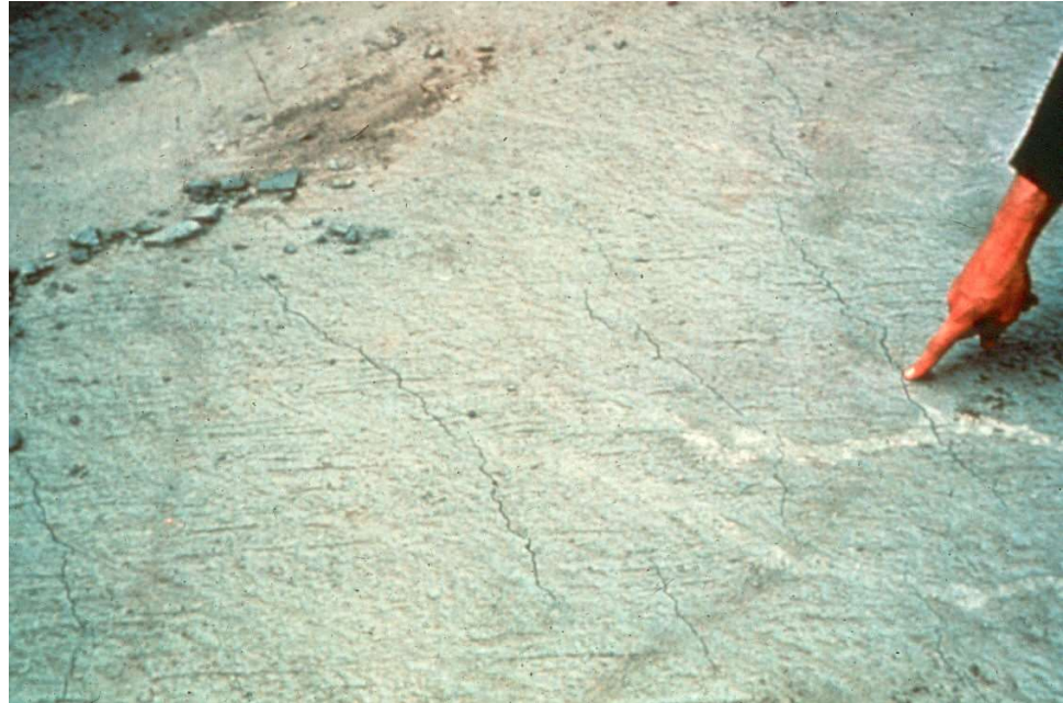
Figure 6.2.15 Temperature Cracks
