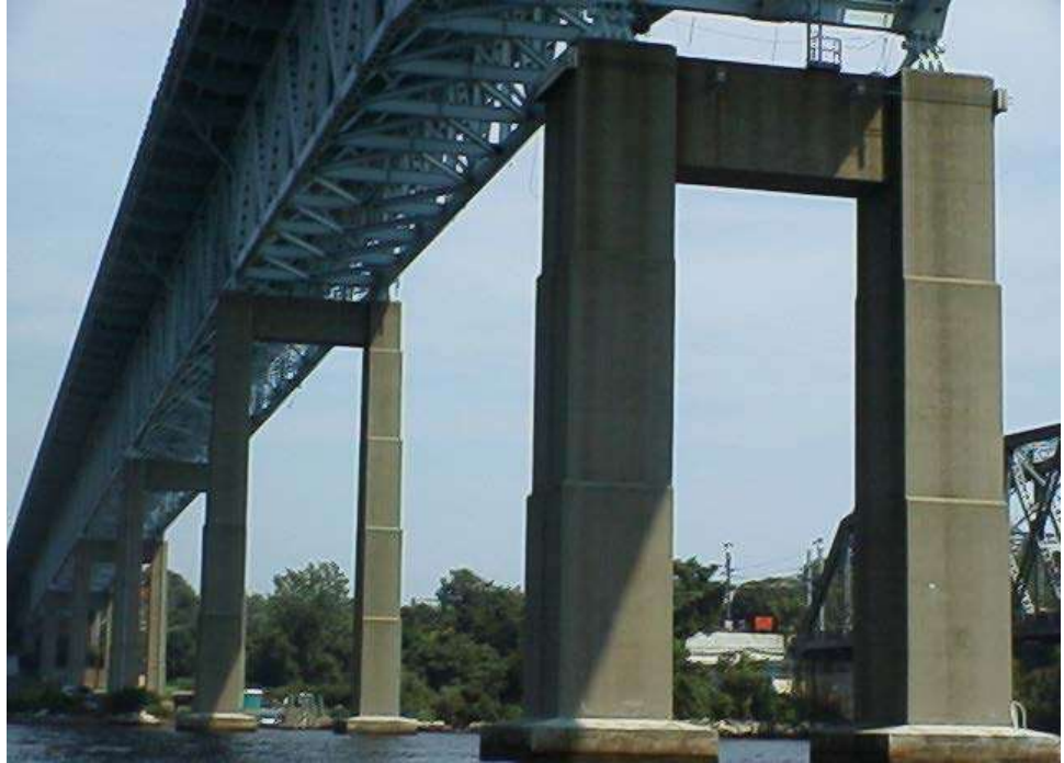
Figure 6.2.2 Rectangular Concrete Members
