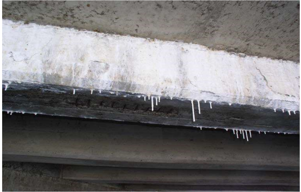
Figure 6.2.25 Efflorescence
