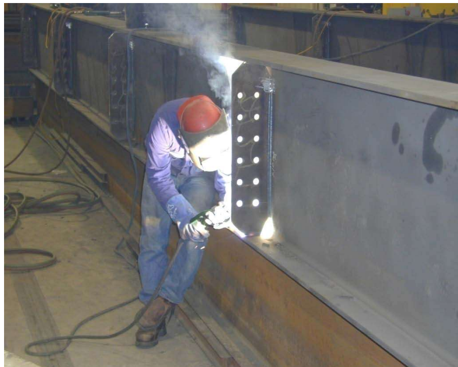
Figure 6.3.3 Steel Plate Welded to Girder
