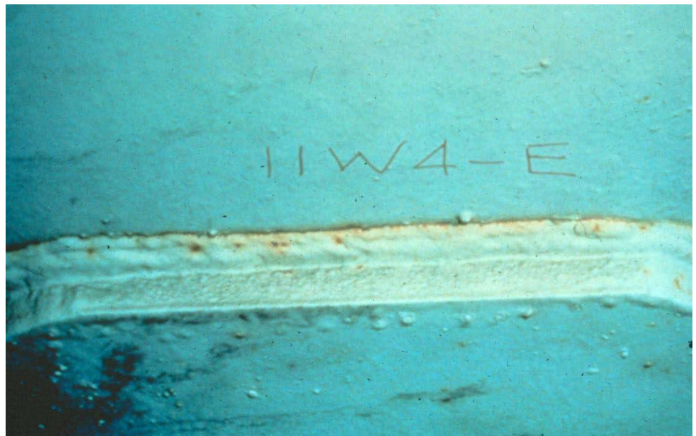
Figure 6.3.21 Fatigue Crack
