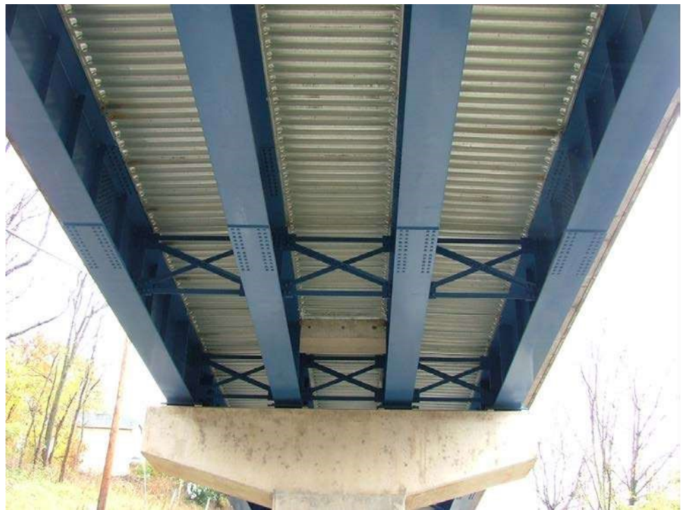
Figure 6.4.4 Load Path Redundant Multi-Girder Bridge
