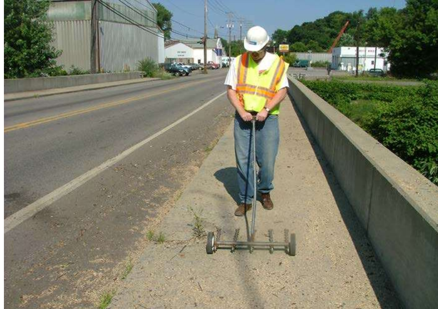
Figure 6.2.33: Inspector Using a Chain Drag
