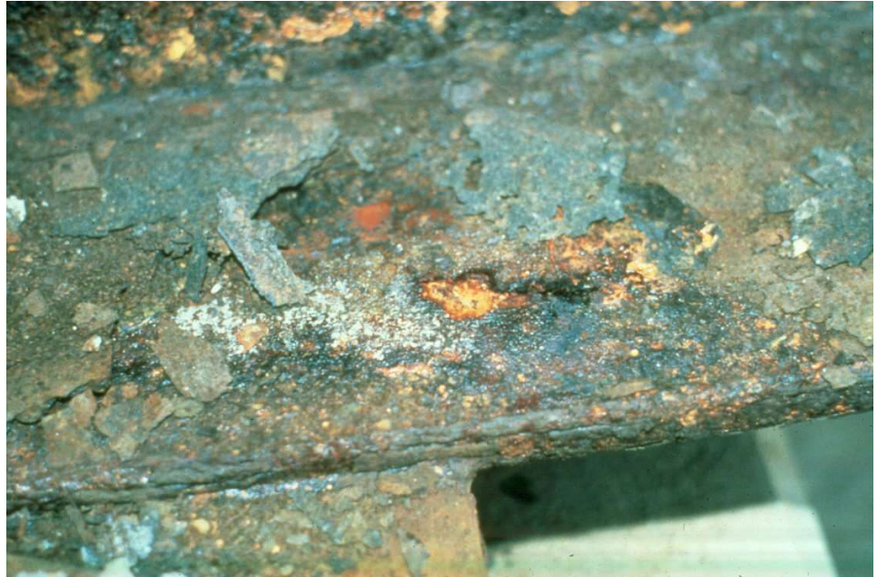
Figure 6.3.26 Color of Oxide Film is Critical in the Inspection of Weathering Steel; Dark Black Color in an Indication of Non-protective Oxide
