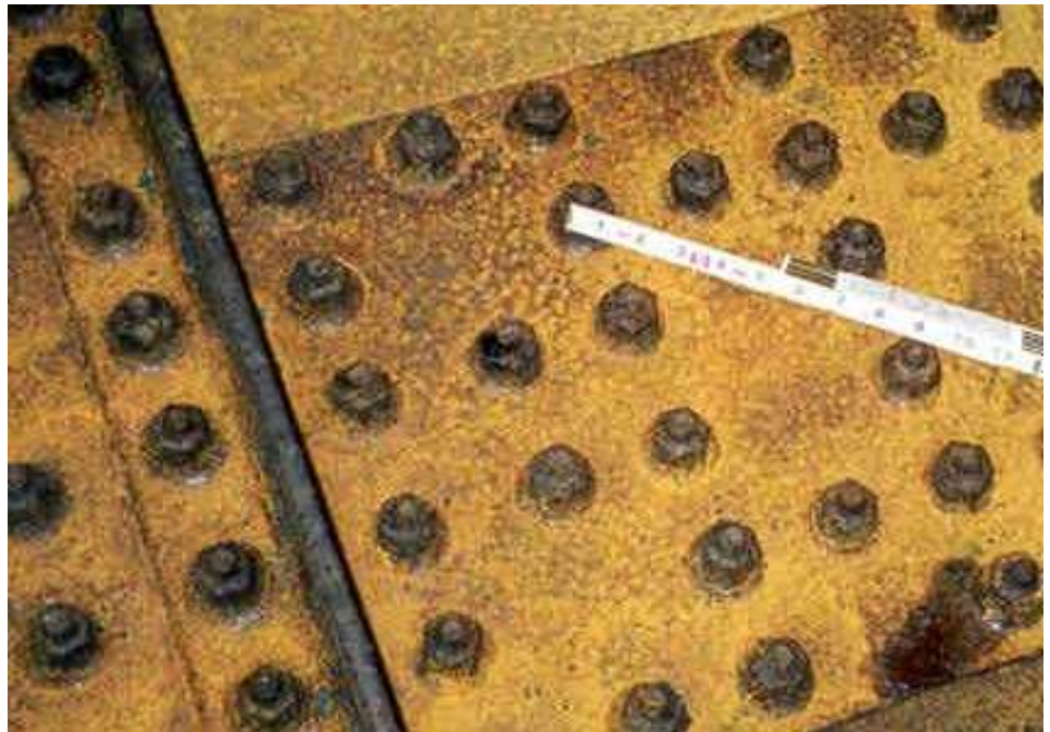
Figure 6.3.27 Yellow Orange – Early Development of the Oxide Film (Patina)
