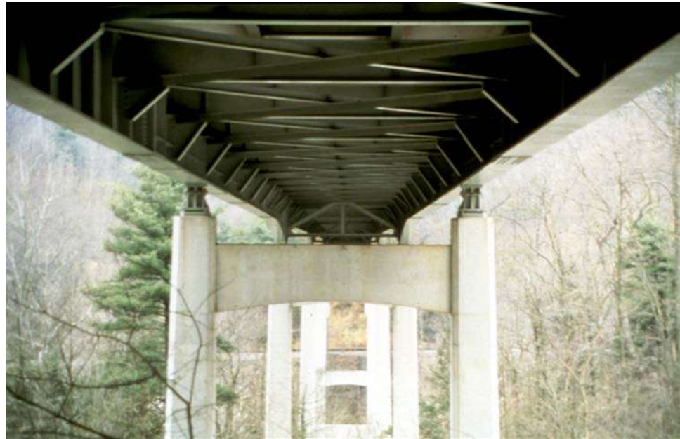
Figure 6.4.9 Non-redundant Two-Girder Bridge
