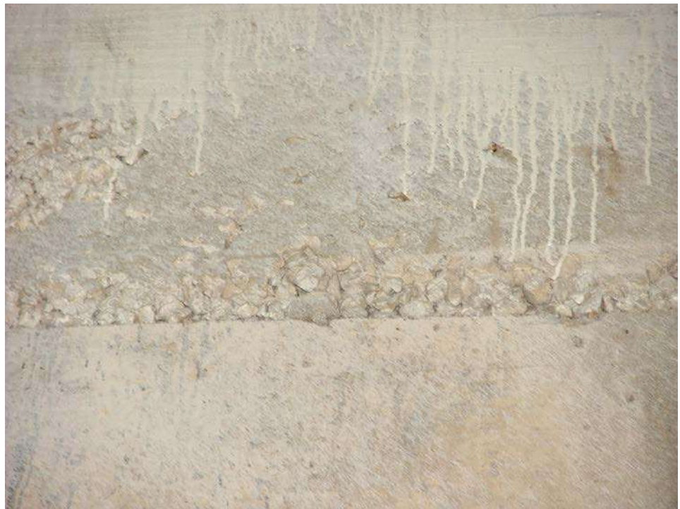
Figure 6.2.27 Honeycomb
