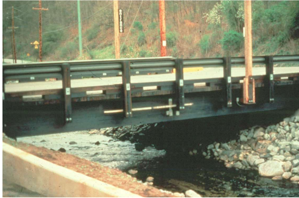
Figure 6.1.1 Glued-laminated Modern Timber Bridge
