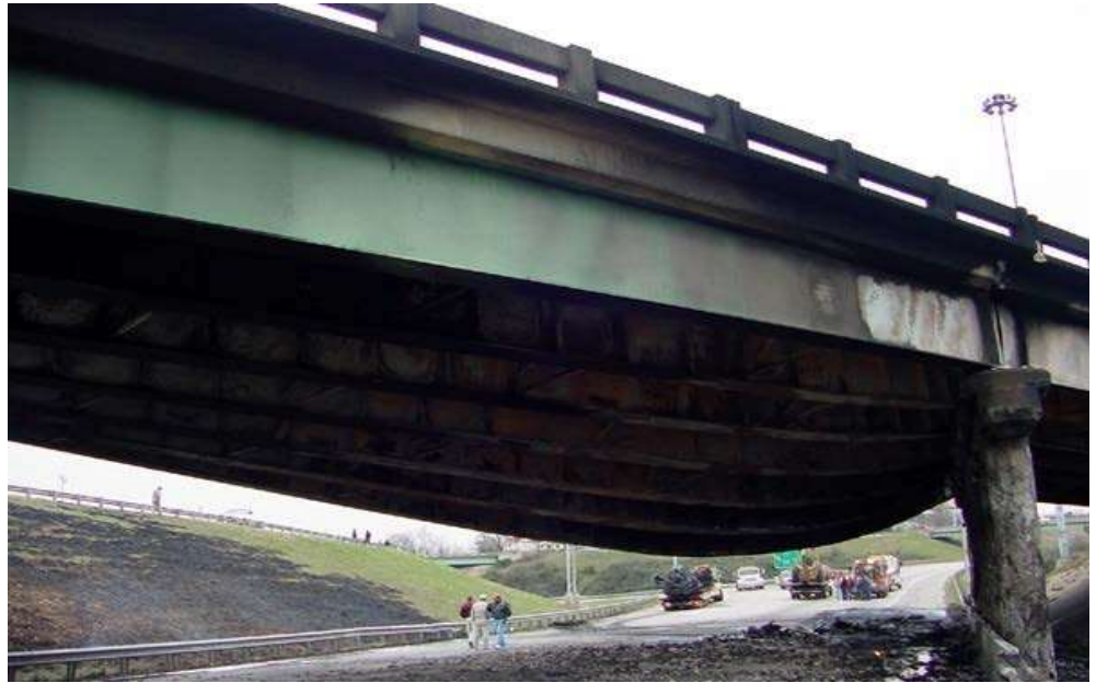
Figure 6.3.14 Heat Damage
