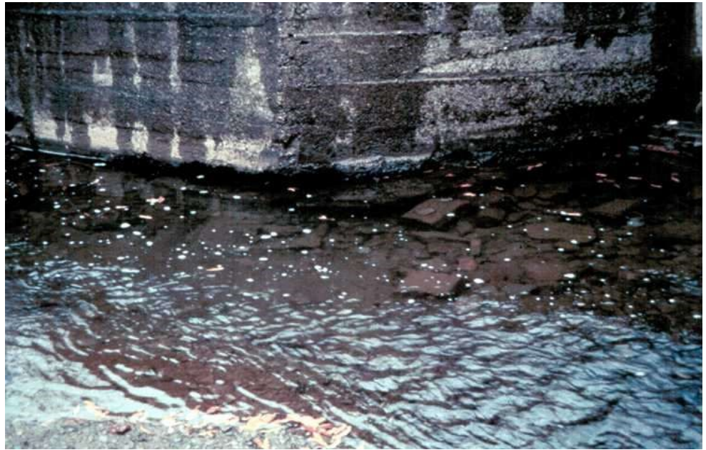
Figure 6.2.29 Substructure Abrasion
