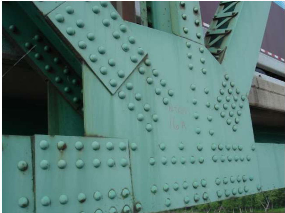
Figure 6.4.44 Riveted Gusset Plate Connection
