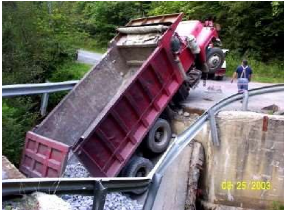
Figure 6.2.30 Overload Damage
