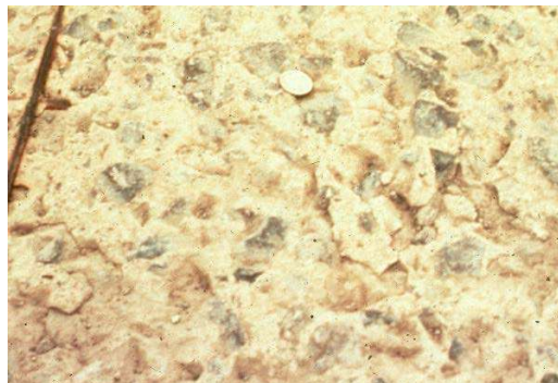
Figure 6.2.23 Severe Scaling
