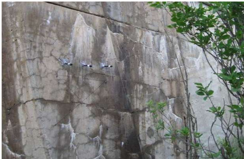
Figure 6.2.26 Alkali-Silica Reaction (ASR)
