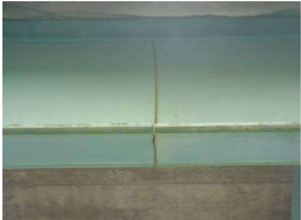
Figure 6.3.11 Fatigue Crack
