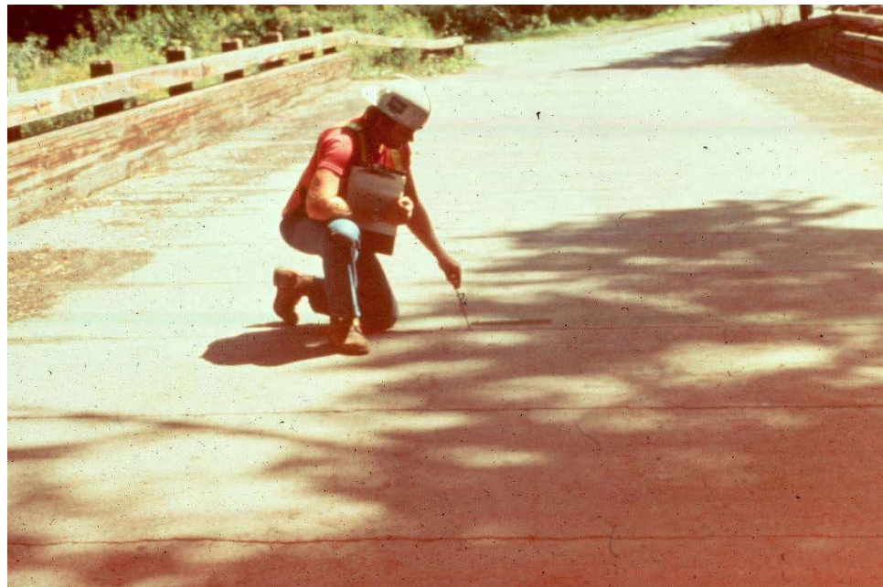
Figure 6.1.29 Inspector Performing a Pick Test
