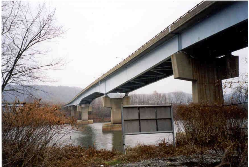
Figure 6.3.8 Built-up Girder
