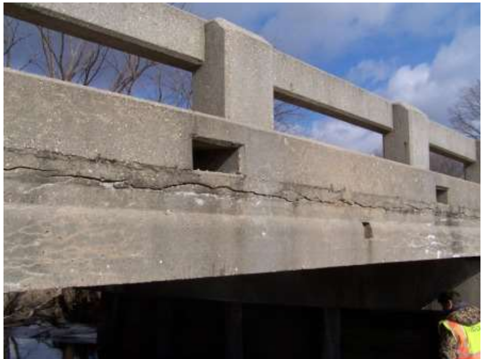
Figure 6.2.18 Longitudinal Cracks
